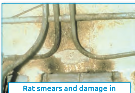
Even metal pipes can be gnawed
