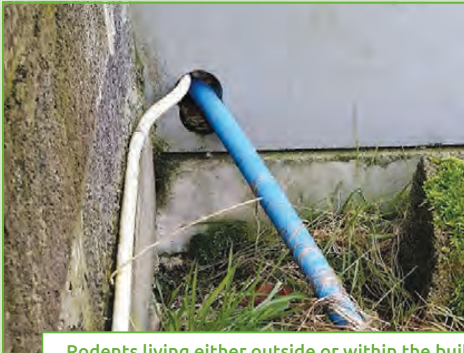
Rodents living either outside or within the building fabric can use gaps around pipes to migrate in and around a building
