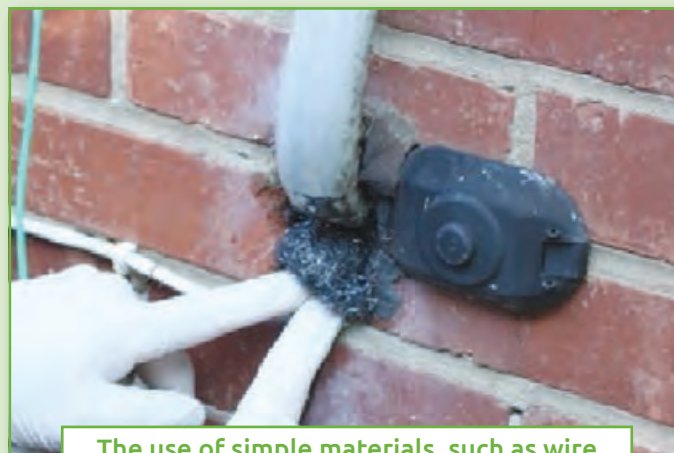
The use of simple materials, such as wire wool, can be very effective to prevent rodent access
