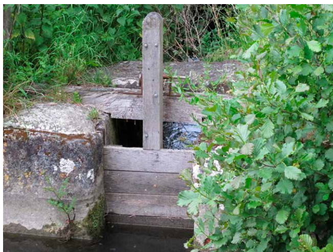
Figure 10 (top) Removing trees, a first step towards conserving sluices, Turnastone Court Farm, Herefordshire.
