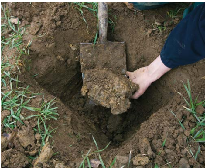
Figure 7. Clay subsoil showing vertical fissuring
