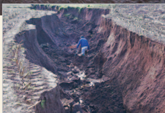
Serious gully erosion
