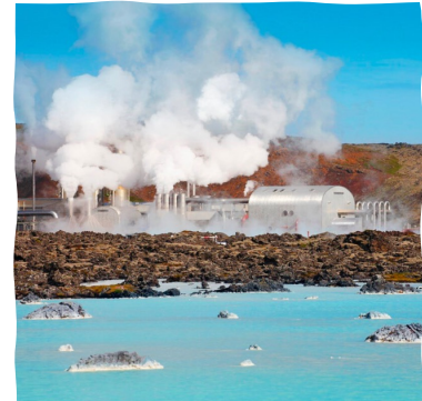
geothermal power plant at Blue Lagoon, Iceland offers an example of how Britain could ease its energy crisis (Getty/Stock)
