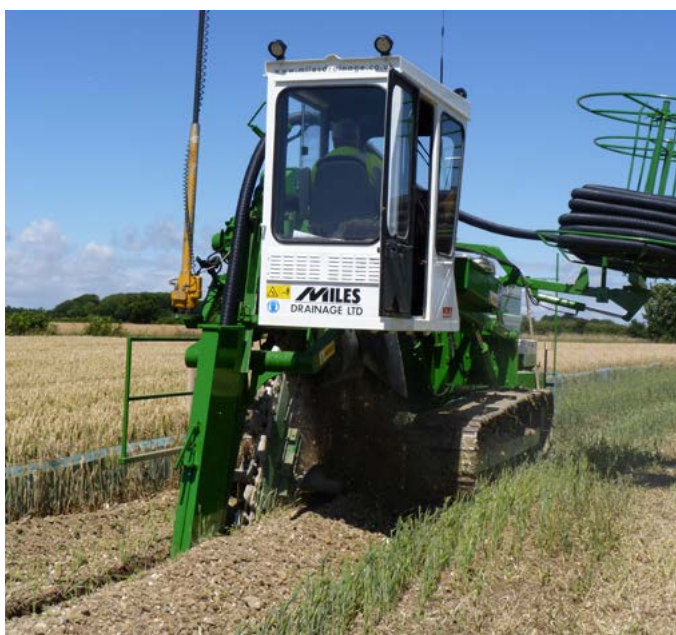
Figure 31. Installing land drains with laser gradient control
